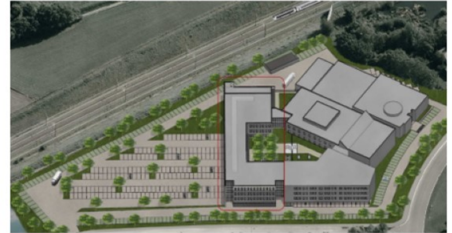
Extension of facility in Belgium
